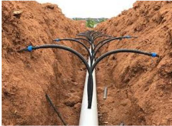
**Figure 6.** Underground irrigation system (URL-4)
